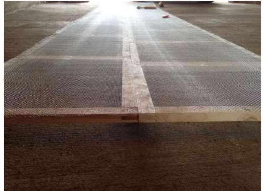
Overlap the covers one half inch per ten feet, staple the ends, remove the half inch overlap, then press both ends down to stretch, and staple the wire to each inner cover frame.
